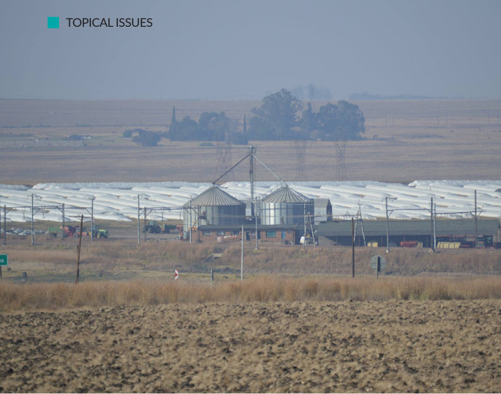
Rising yields led to the adoption of bunker storage and silobags as practical alternatives to constructing new silos. (Photograph: Silostrat)
