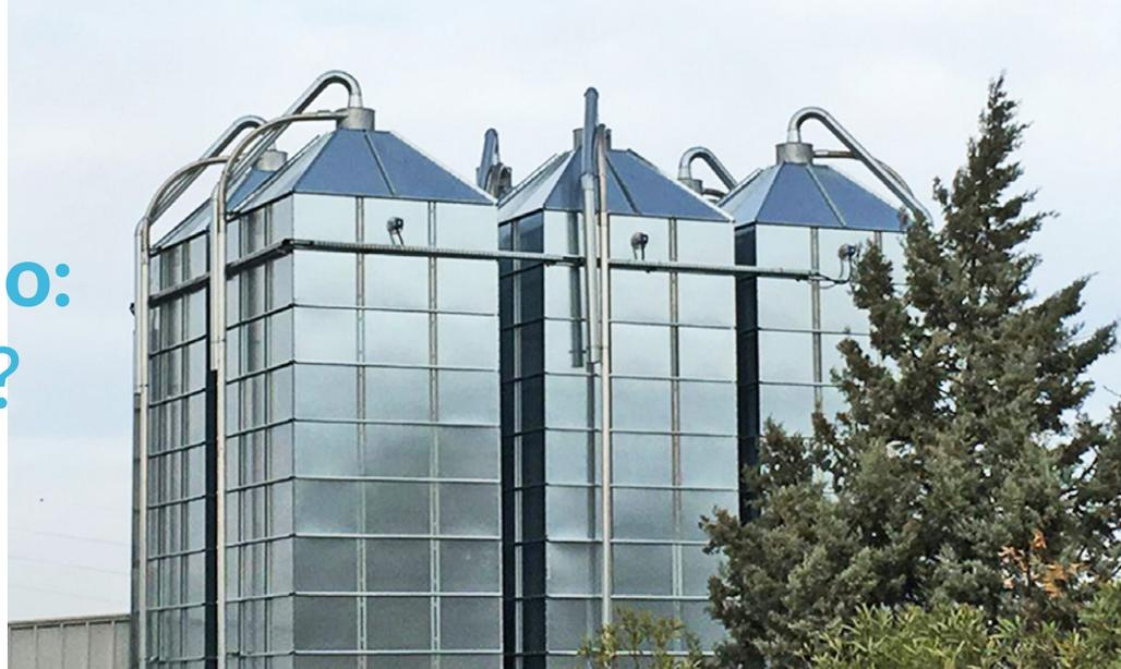
A set of square silos constructed by Indian company, Invoit. (Image: [www.invoitplast.in/square-silos/](http://www.invoitplast.in/square-silos/))
