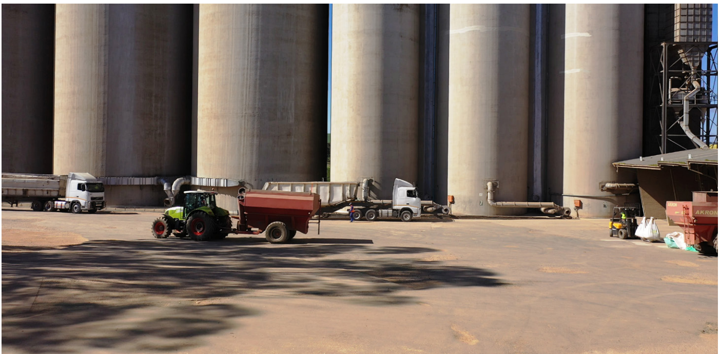
The Overberg Agri Rietpoel silos. (Photograph: Overberg Agri)
